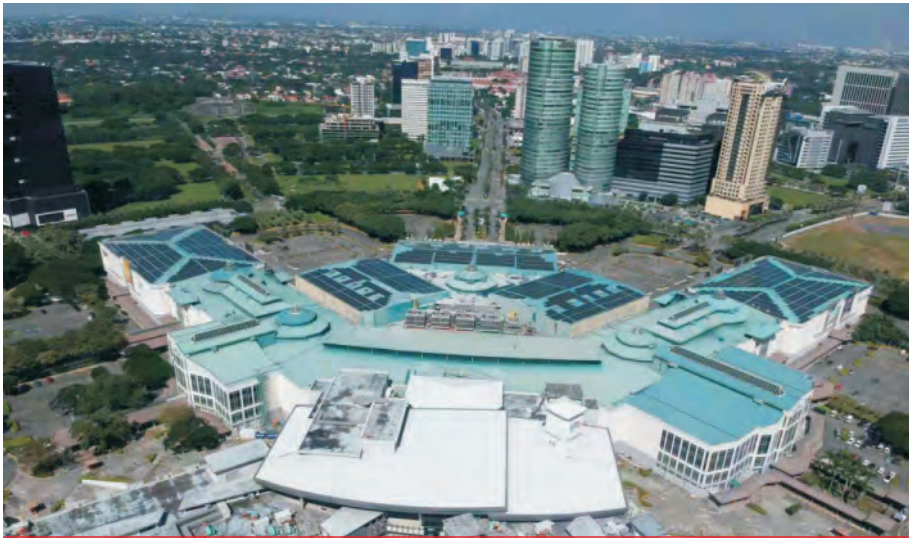
CASE STUDY: Festival Supermall Alabang Solar Rooftop, 2.8MW
