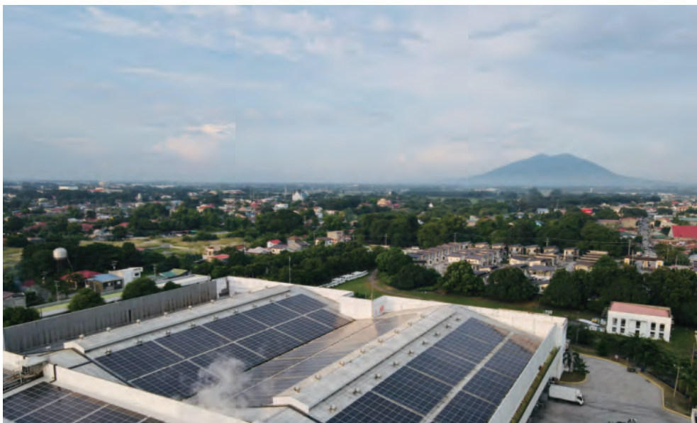
CASE STUDY: Pampanga, Philippines 1.3MW
