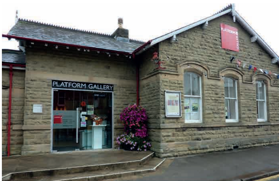
EndoTherm™ was trialled at the Platform Gallery by Ribble Valley Borough Council
