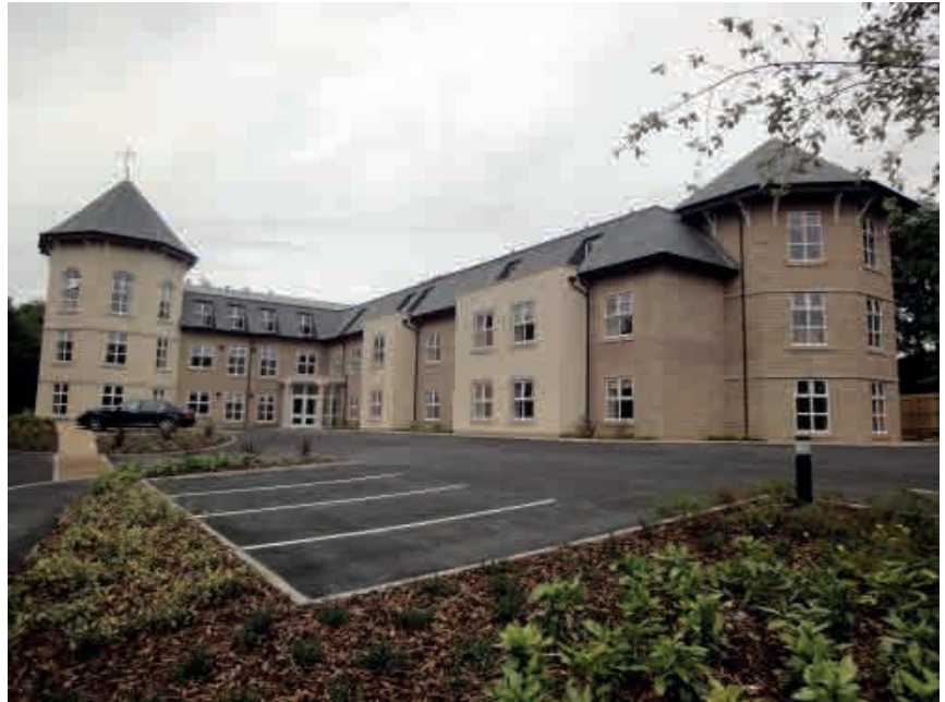
EndoTherm™ was trialled at Nelson Manor Care Home in Nelson, Lancashire
