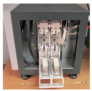
Figure 4-13: battery storage system, side view, power isolator pulled
