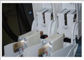
Figure 4-8: representation of the correctly inserted fuses
