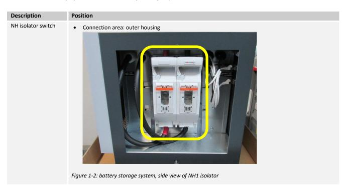
The externally accessible fuse elements (NH1) ensure the line protection and short-circuit protection.
