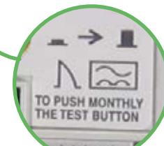
Type A: Tripping is ensured for residual sinusoidal AC in the presence of residual pulsating DC.
